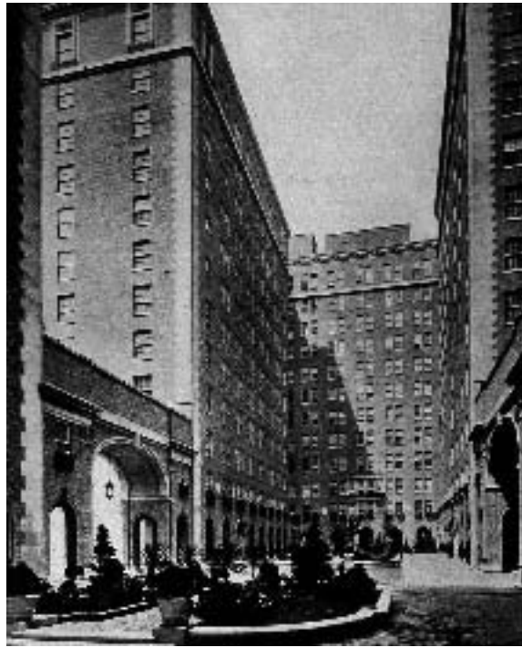
Fig. 74: Wetmore and Warren, apartment block at Park Avenue in New York, 1918.
