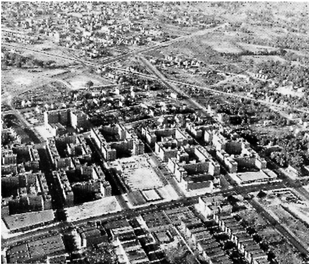
Fig. 77: Clarence S. Stein, Hillside Homes at the Bronx in New York, 1932-35.
