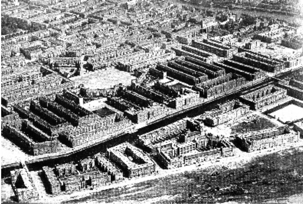
Fig. 32: Hendrik Petrus Berlage, Pieter Lodewijk Kramer, Michel de Klerk and others, urban neighbourhood at Amsterdam-South, 1917-23.
