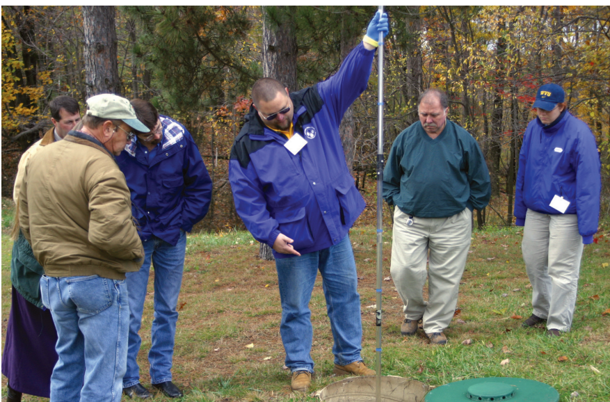
Figure 13: Using a “sludge judge” to inspect solids accumulation in a septic tank.
