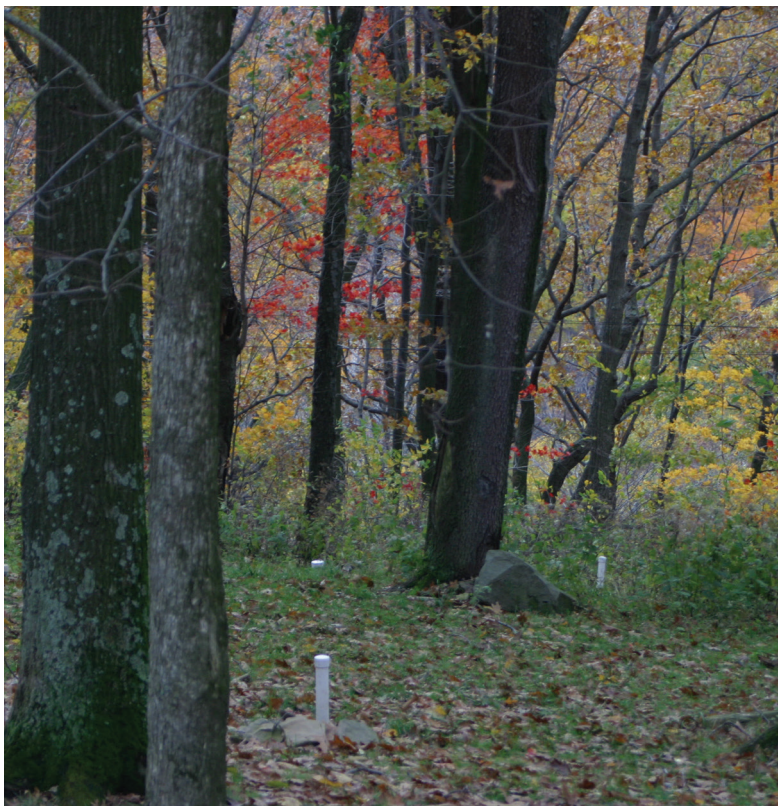
Figure 11: LPP system in ground, showing inspection ports.
